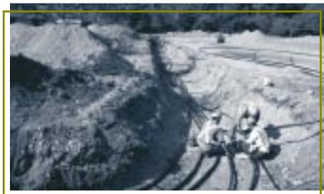
Groundwork following a \$1 million investment in energy conservation measures involved more than installing ground source heat pumps, pictured above, in two Coquitlam, BC schools. The district also set up an energy monitoring and management system that includes documenting GHG reductions through VCR progress reports. It hopes to sell its reduction in a future emissions trading scheme.
