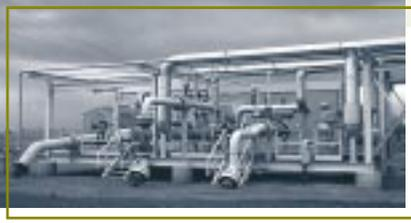
At the end of a 325-kilometre pipeline, crossing the border from North Dakota, CO<sub>2</sub> arrives at this inlet skid in the EnCana plant yard in Saskatchewan. Injecting the CO<sub>2</sub> into its Weyburn oilfield, EnCana is boosting petroleum production while reducing greenhouse gas emissions.
