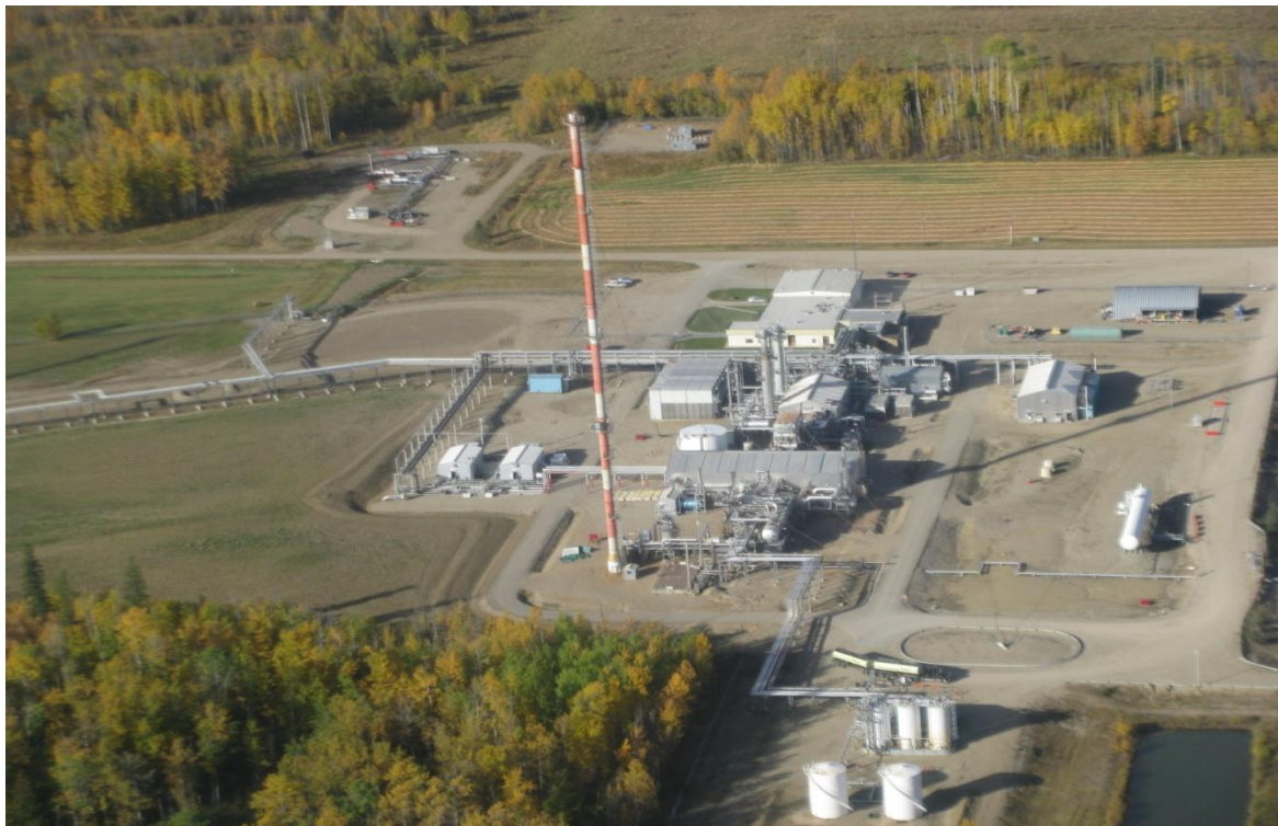
Figure 1-1 : Bonavista South Rosevear Gas Plant
